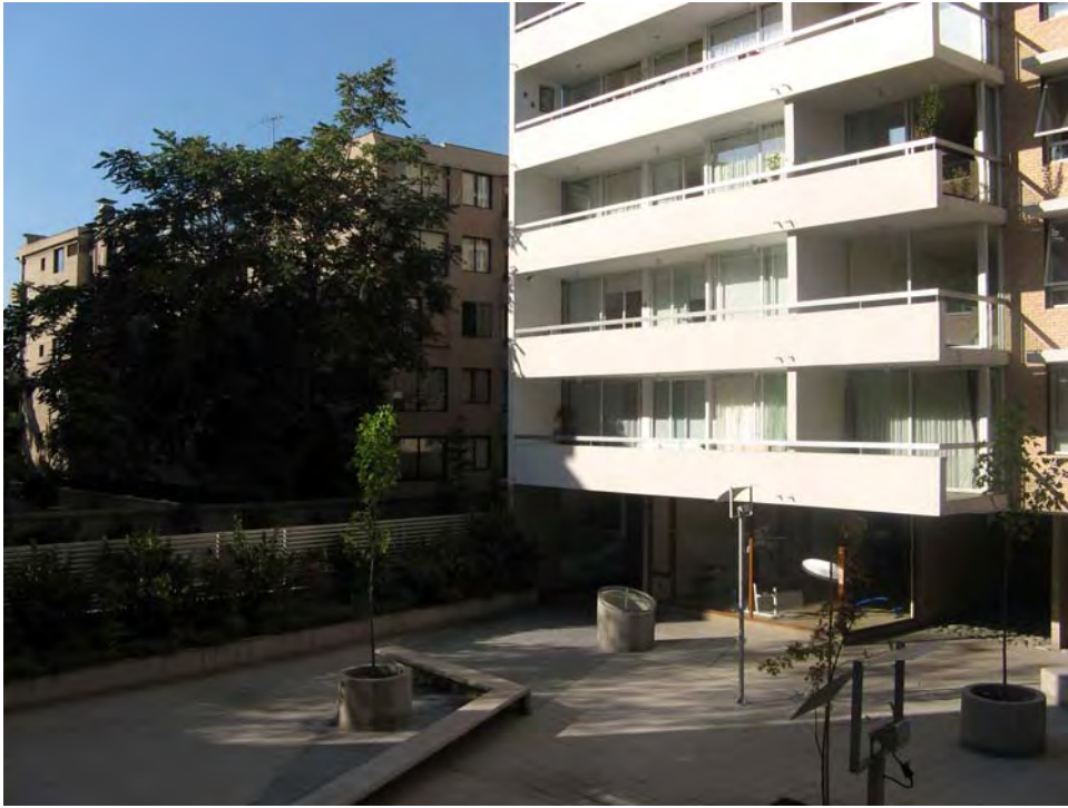
Figure 7-7. This image shows the photograph taken with the automatic settings of the camera for reference.
